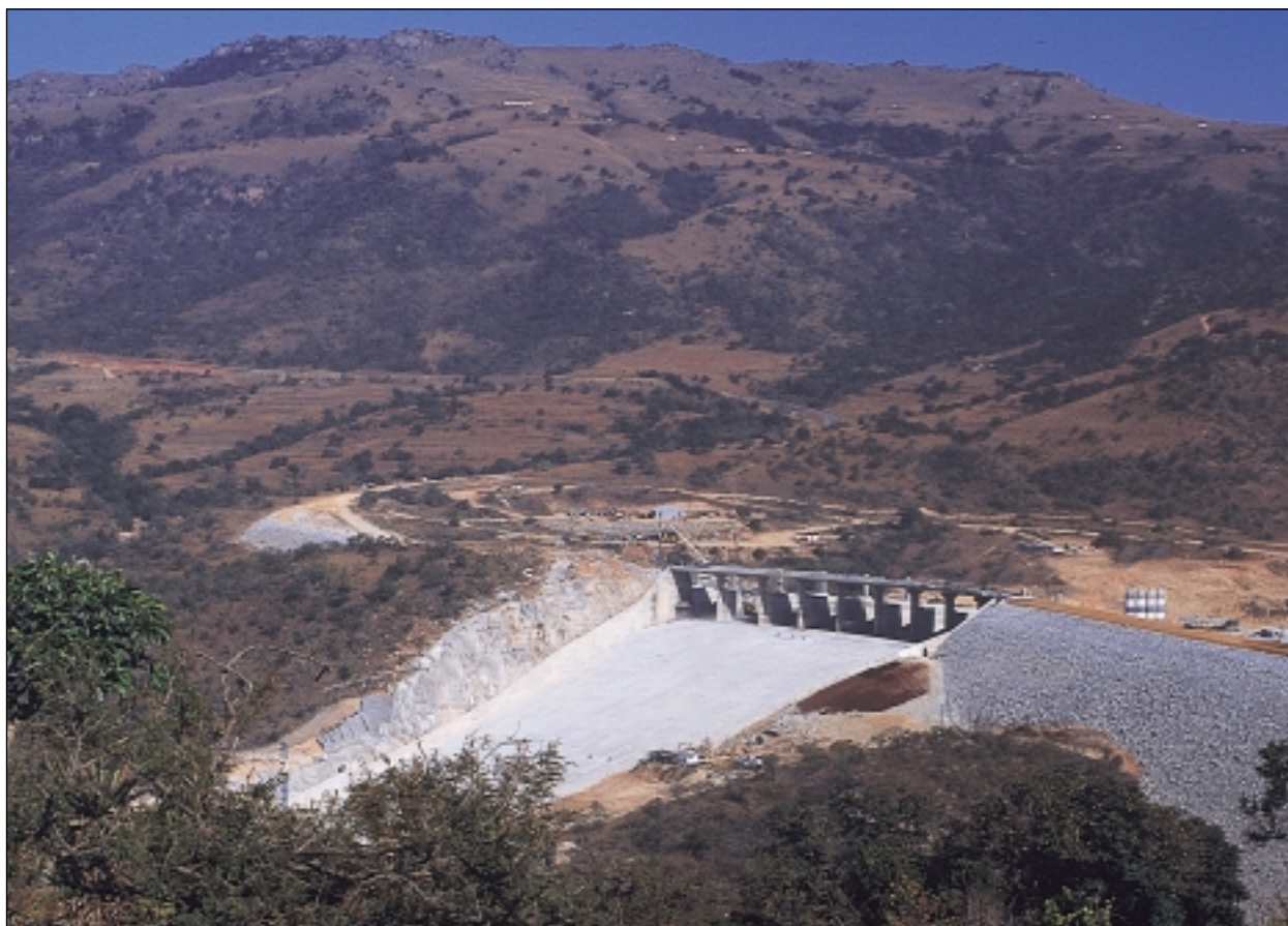
Dam construction site over the Komati River (Maguga Dam)
