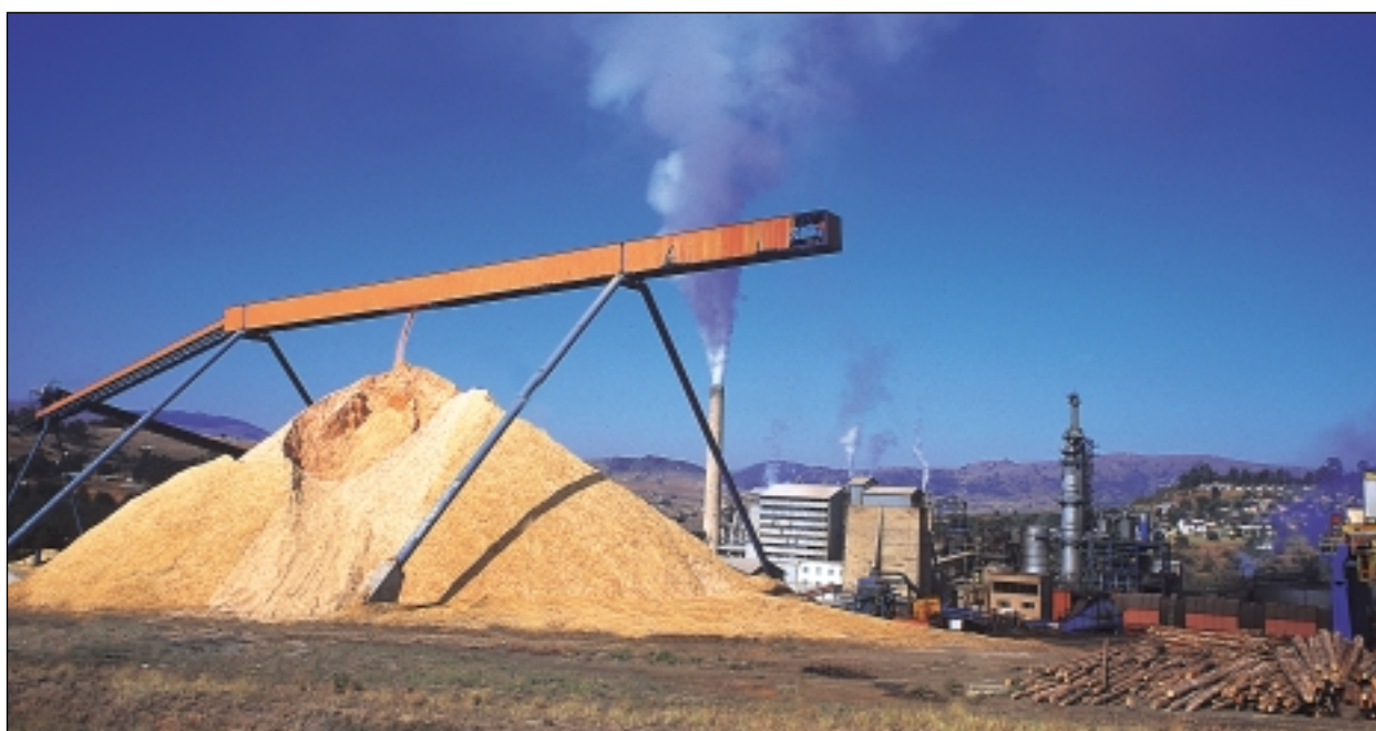
Pulp mill at Bhunya with wood chip stockpile
